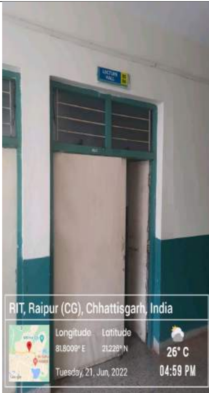
BS06 A Classroom front view LCD Projector with WiFi facility
