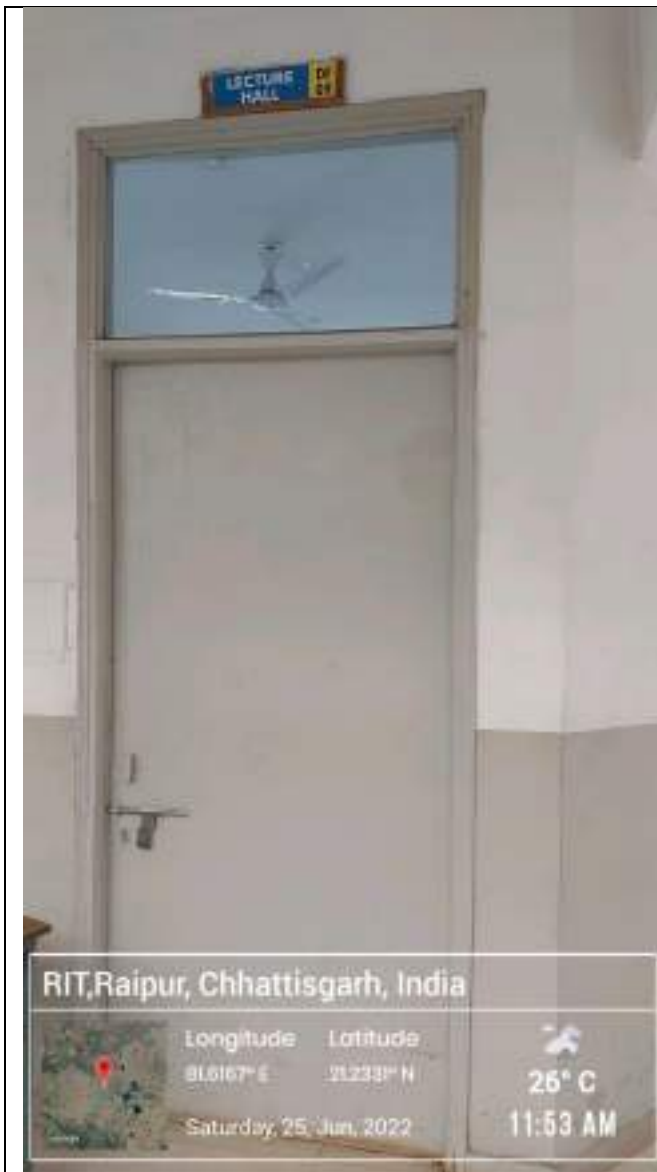
DF09 A Classroom front view LCD Projector with WiFi facility
