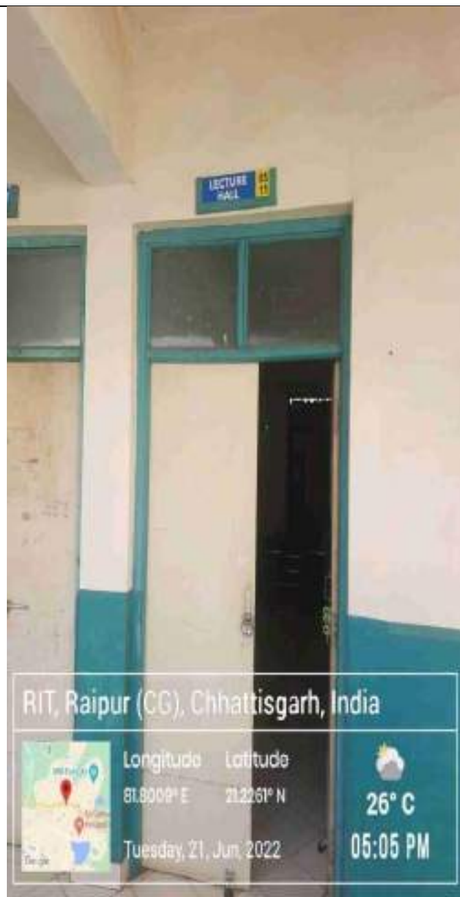
BS11 A Classroom front view LCD Projector with WiFi facility
