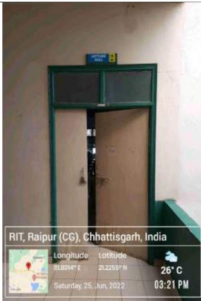
CS01 A Classroom front view LCD Projector with WiFi facility
