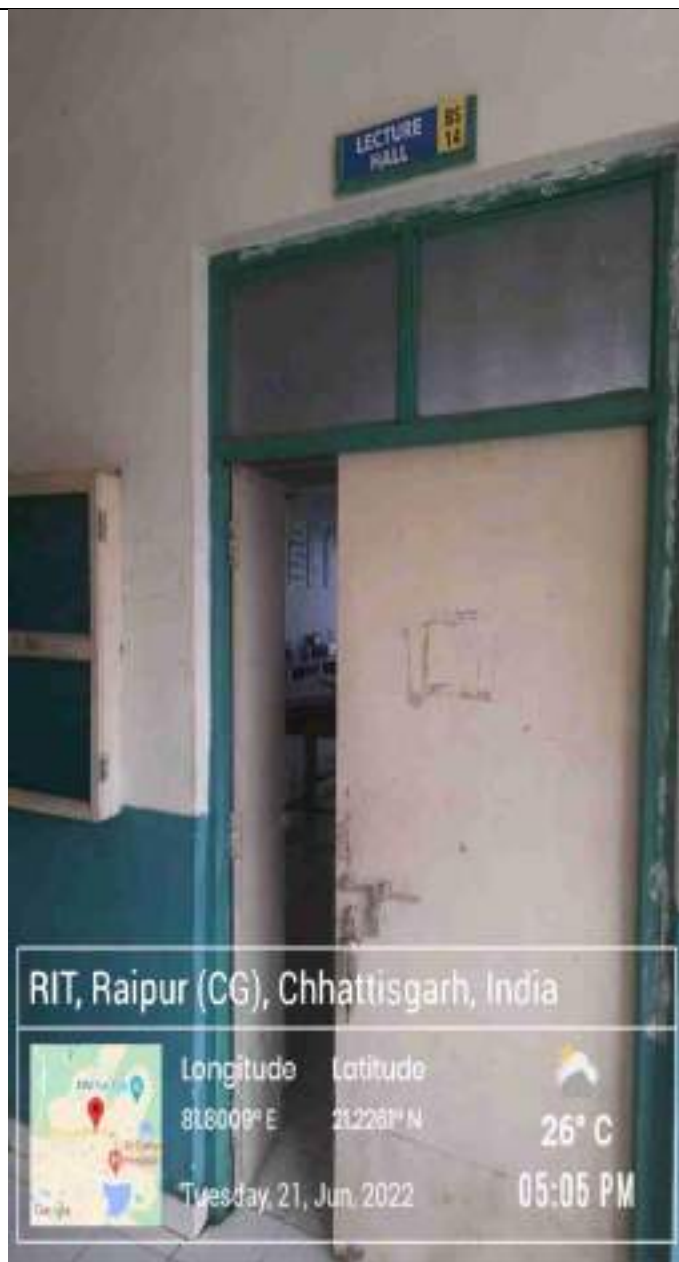
BS14 A Classroom front view LCD Projector with WiFi facility
