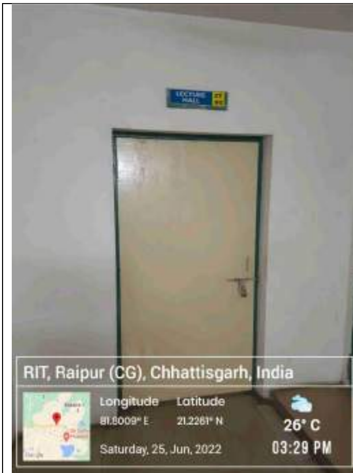
CT02 A Classroom front view LCD Projector with WiFi facility
