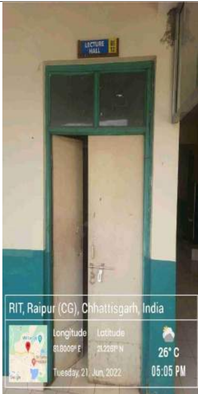
BS12 A Classroom front view LCD Projector with WiFi facility
