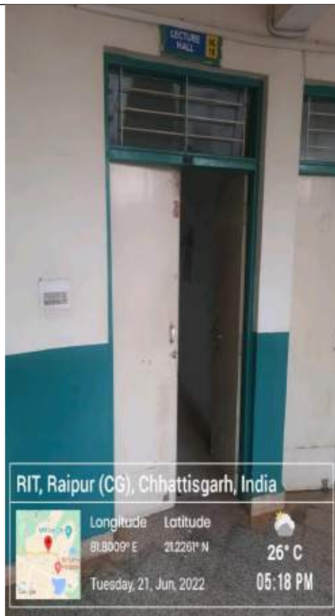
BG10 A Classroom front view LCD Projector with WiFi facility
