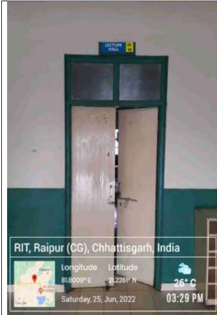
CS18 A Classroom front view LCD Projector with WiFi facility
